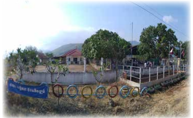
External View of Pailin Church & Primary School
